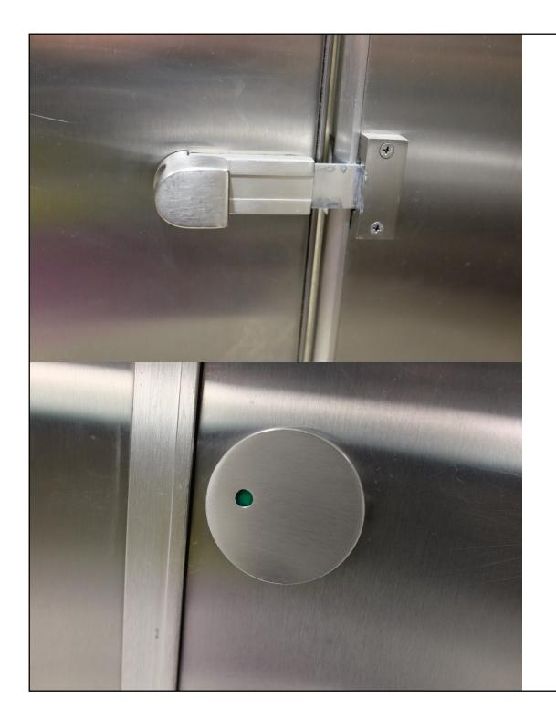
Locking and unlocking door automatically changes color of lock indicator
